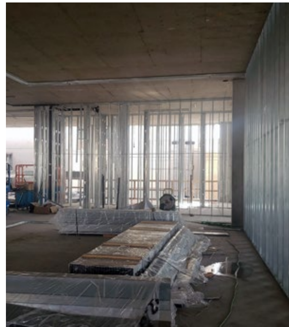
Framing on the ER gets underway at Peace Arch Hospital.
